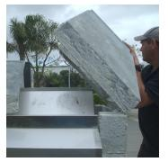
**10.** Position and glue the two Chimney Gathering Blocks on top of the visor and Outer Firebox as shown.
