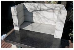
**3.** Build three layers of the Outer Firebox, gluing each layer as you go. The rough edge faces up (opposite way up to the Woodbox).
