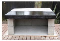
2. Place the plain concrete mantle/hearth flush with the rear of the Woodbox and the polished & UV sealed mantle/hearth with the display edge facing outwards. Check for level before gluing in place.
