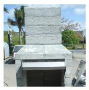
11. Place and glue the Chimney Blocks one on top of the other ensuring they remain straight and level as you go.
