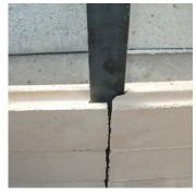
6. Build the back wall of the Inner Firebox, placing the two larger blocks first with the steel forming bar in the centre. The shorter side of the forming bar is the bottom. To get the blocks to fit nicely, use a grinder to clean out the inner groove and remove rough edges on the outer wall side.
