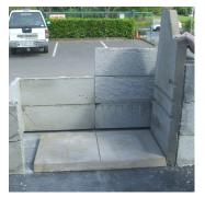
Locate the Inner Firebox Base (large rectangular piece with sloped front edge). Using your grinder, cut a 5mm deep controlled crack line across the middle. Begin placing the firebox components as shown.
