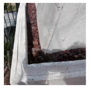
8. Make sure your Inner Firebox Side Walls are parallel and the back wall fits tightly then fill the cavity between the inner and outer firebox with 120L of Scoria 25/7.
