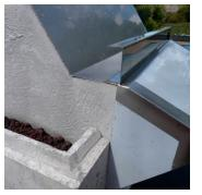
Fit the stainless steel visor ensuring you align with the contours of the firebox sides then build the fourth layer of the Inner Firebox. It is important to check for level here.
