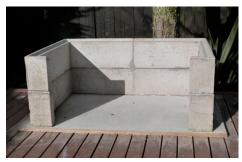
1. Place Woodbox Blocks (large "L" sections) on foundation as pictured. The two blocks with the flat base go on the bottom. Apply Gorilla Grip along all edges and joins.
